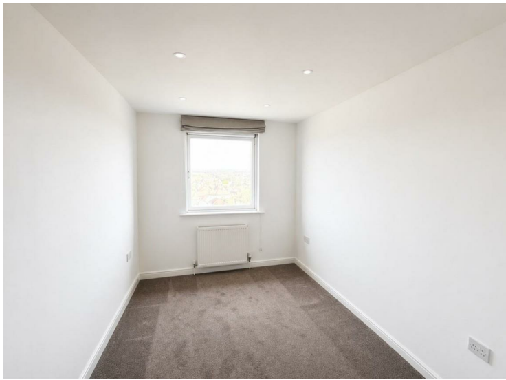
Rear aspect double glazed window, electric heater.
